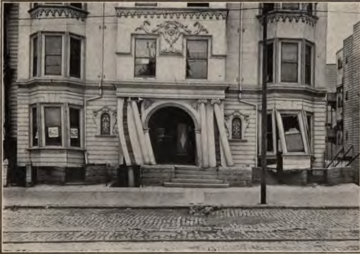
A. House which slid upon its foundation a distance of four feet.
